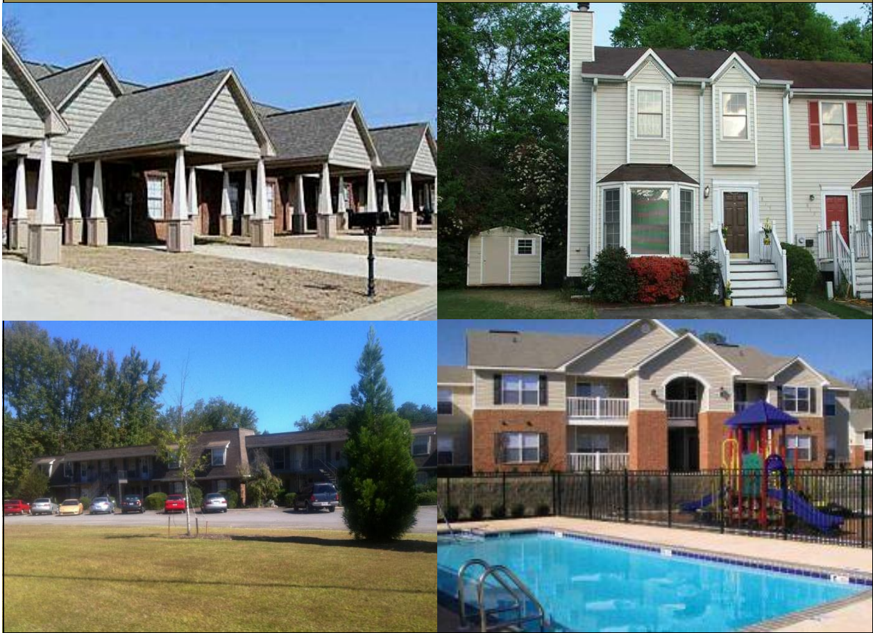
Figure 9.4 High Density Residential Character
